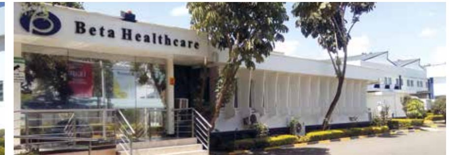
The newly refurbished entrance and reception area of the administration block.
